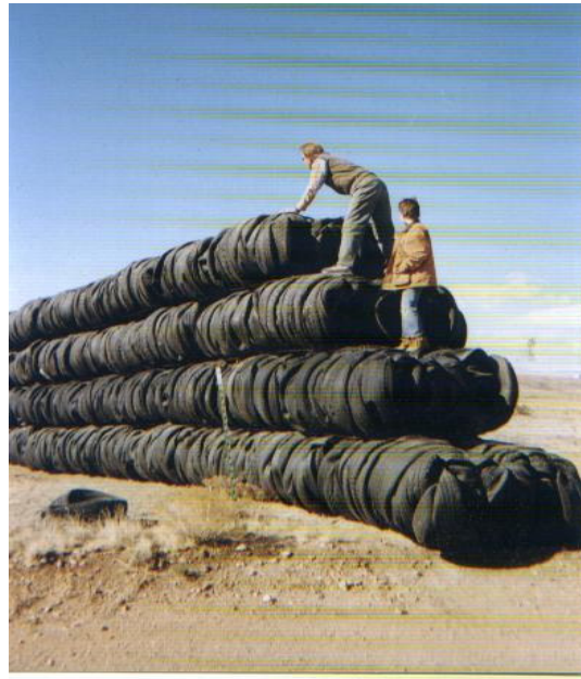
Figure 4 – Four-High Bale Wall
