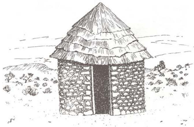
Figure 1: A rondavel built of earth and stone
