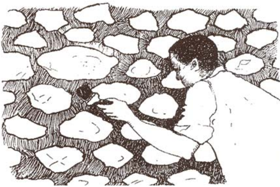
Figure 8: Brushing the joints with clean water must be done after each day's work.
